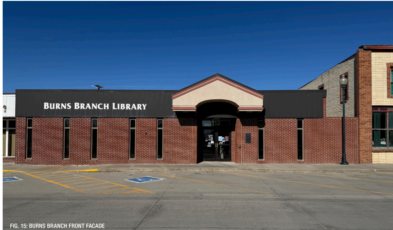
FIG. 15: BURNS BRANCH FRONT FACADE
