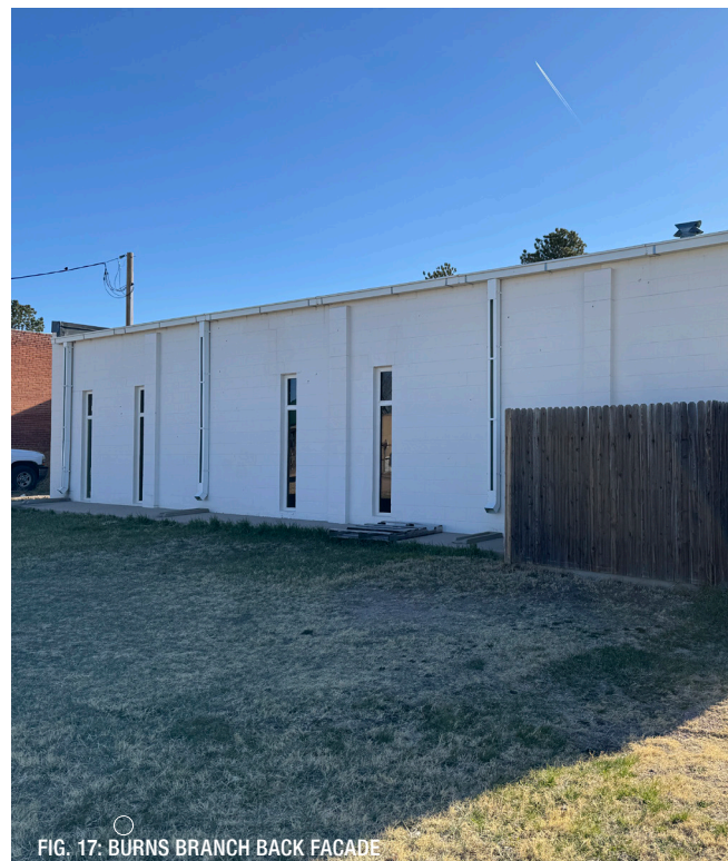
FIG. 17: BURNS BRANCH BACK FACADE
