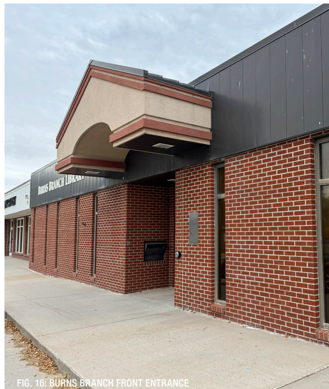
FIG. 16: BURNS BRANCH FRONT ENTRANCE
